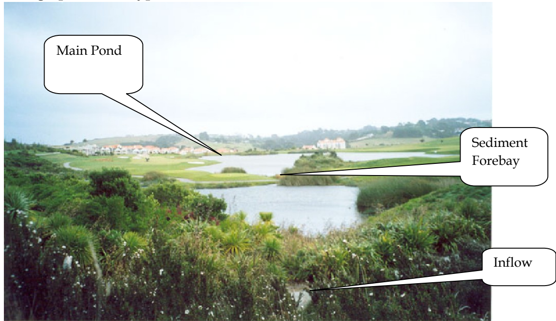
Photograph 1.1: A Typical Stormwater Treatment Pond
