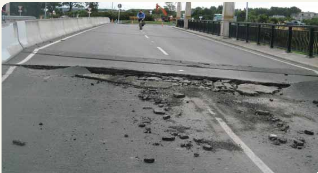
Quake damage to the ANZAC Drive Bridge.
