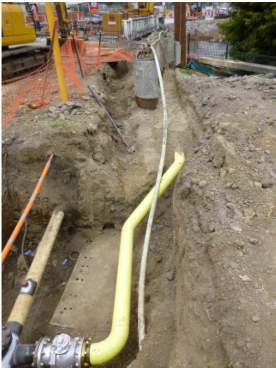
Gas main diversion on the new Wairau Creek Bridge.
