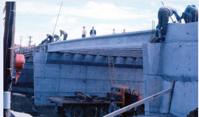
Gladstone Road rail overbridge under construction (Auckland Libraries Heritage Collections 255A-35024).
