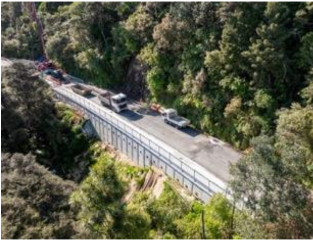
RP0.85 Scenic Drive Titirangi (Piling completed – back filing and drainage underway)
