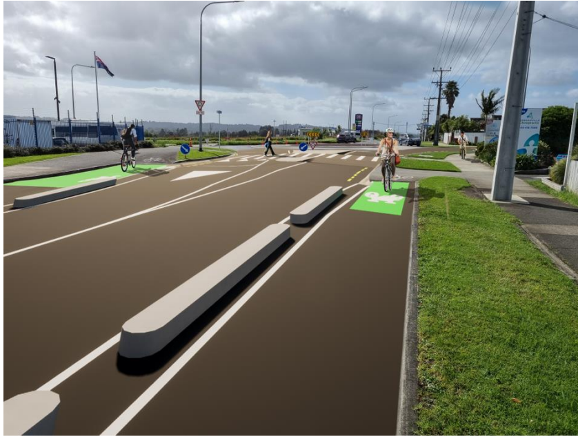
Artist impression of proposed cycleway featuring cycleway separators, one of the proposed options.
