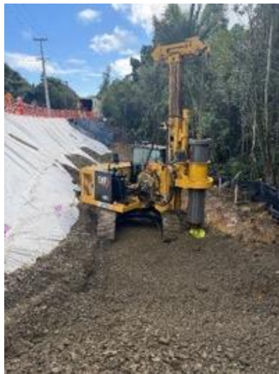
Slip repairs underway on Te Henga Road, Piling works starting
