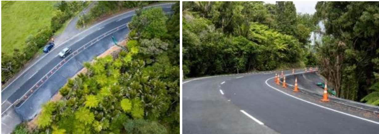
Wairere Road slip site 349 Wairere Road almost complete
