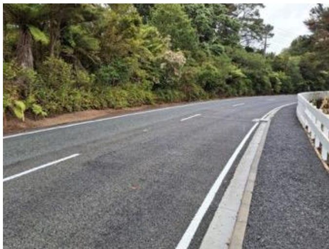
Repair of Simpson Road, outside 163 Simpson Road.
