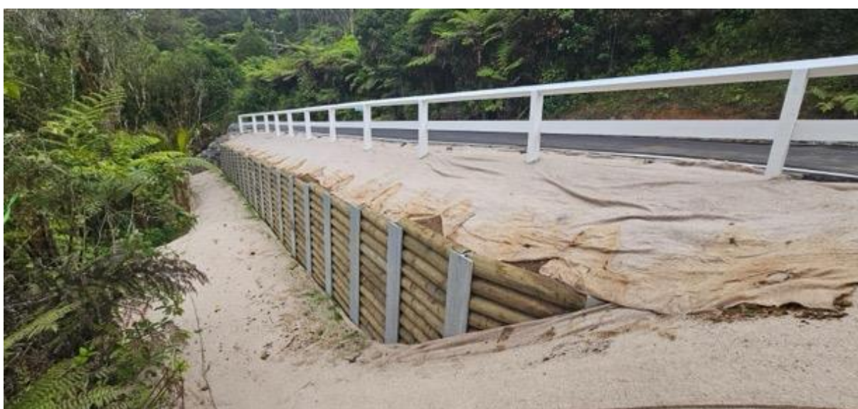
Slip Repairs complete on Kellys Road, Oratia, 9 December 2024.
