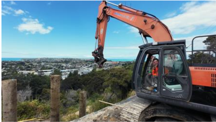
Wade River Road – Retaining Wall construction/ drainage repairs
