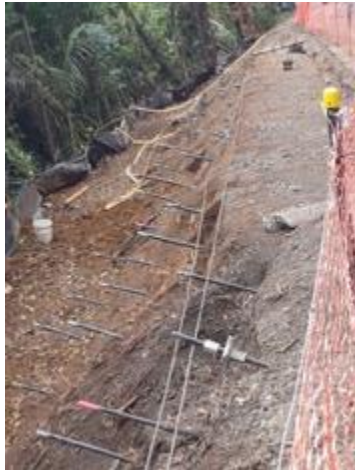
Site RP0.899 Mountain Road – image shows the soil nails that have been installed in January.
