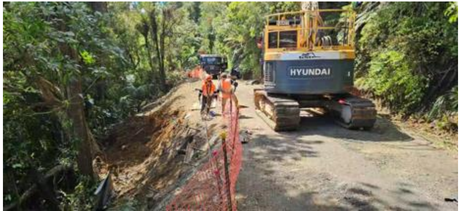
Site RP0.899 Mountain Road – image shows the soil nails that have been installed in January.
