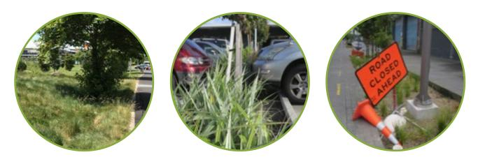
**Left** – The selected turf species allows use of reduced-mowing which improves tree pit and swale bioretention performance and improves tree health (Albany); centre – narrow swale with no car bumpers allows cars to damage plants (Nelson).
