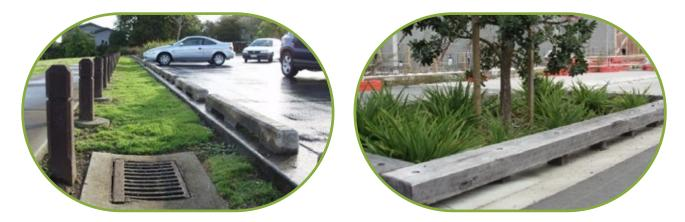
**Left** – The many intruding posts on the left create high maintenance, exacerbated by the use of turf rather than a perennial groundcover and low mowing height reduces efficacy of filtration (Mount Albert).
