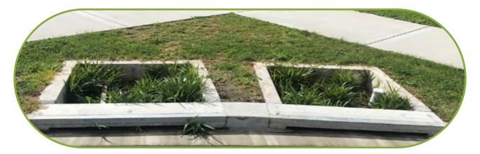
**Low maintenance plants** (an Australian Dianella) placed in device layout that increases maintenance due to the long length of edges. A better design would remove the narrow grass strip by placing the devices together, or use one, larger device (which would also reduce the volume of concrete).
