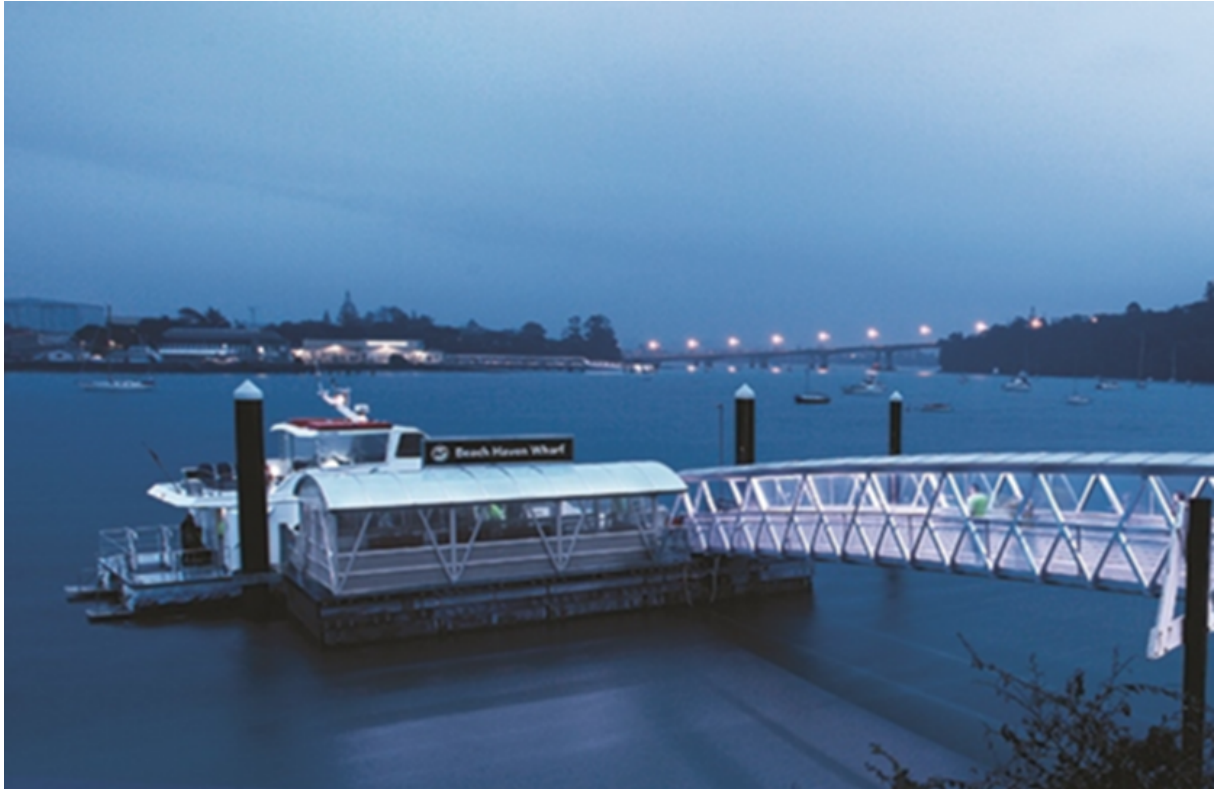
Figure 2-2: Beach Haven wharf – the pontoon structure provides shelter and seating for ferry customers
