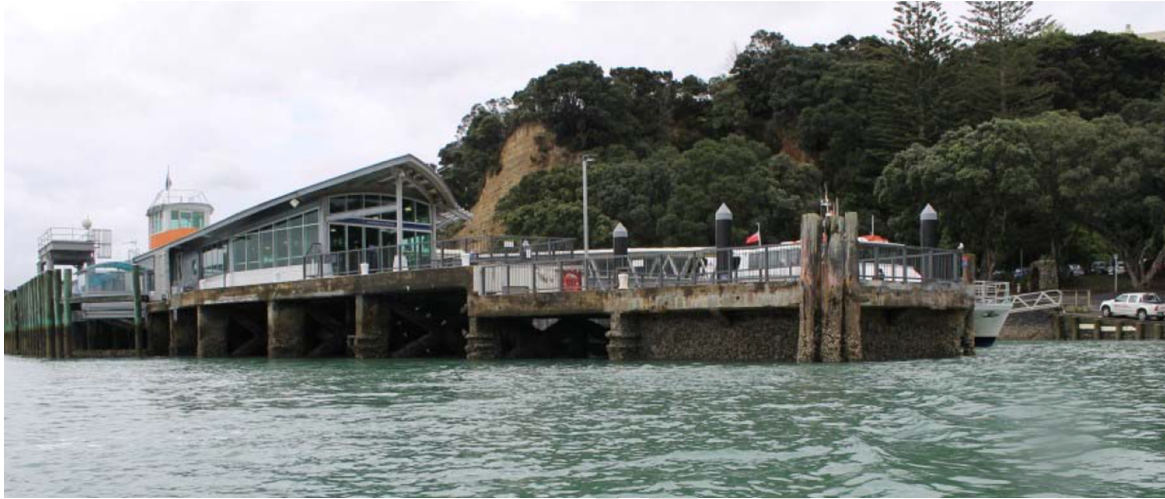
Figure 1-3: Birkenhead wharf and ferry building
