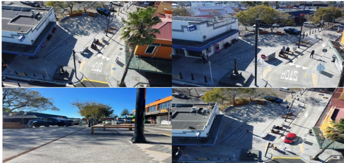
LOCAL BOARD PROJECTS - Criterion Square, Otahuhu work completed
