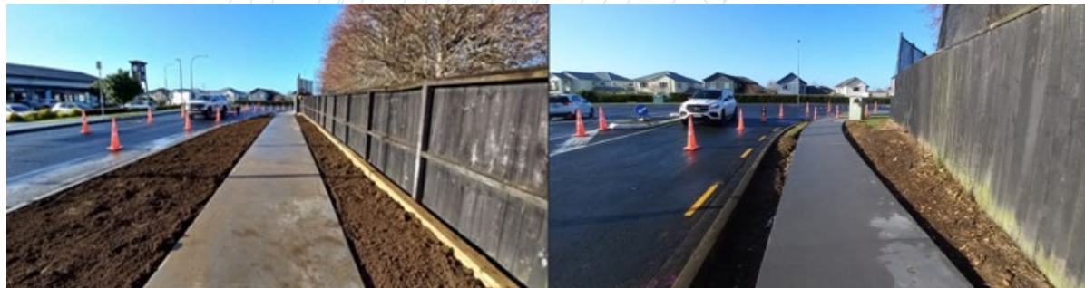
NEW FOOTPATHS: Pararekau Road, Karaka – work in progress
