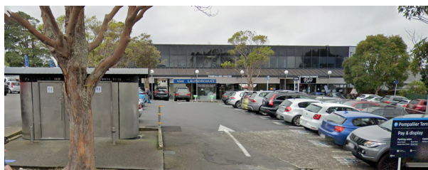
Figure 4: Pompallier Terrace carpark
