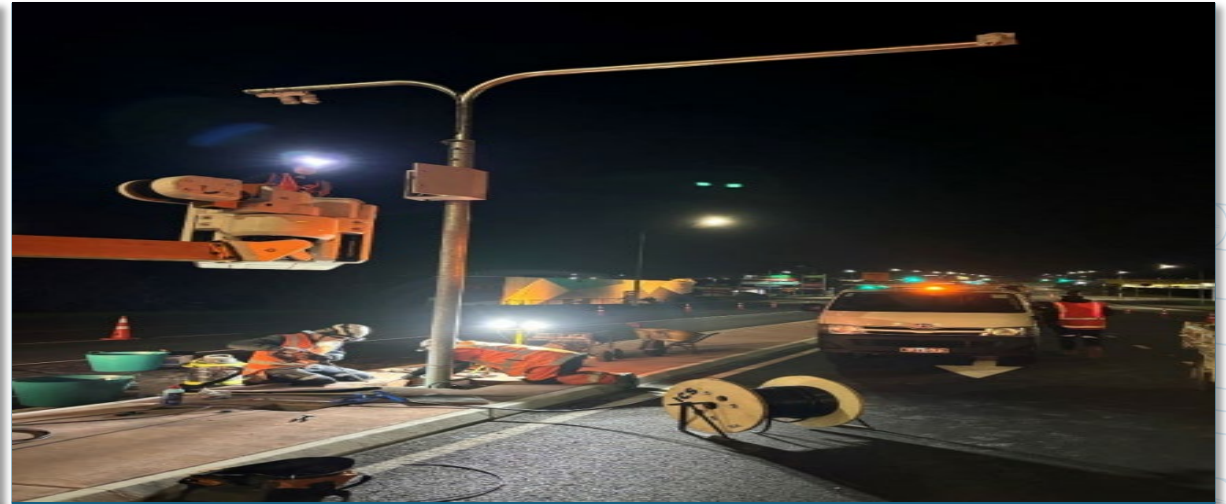
Installation of bus lane camera poles and ducting – Fred Taylor Drive
