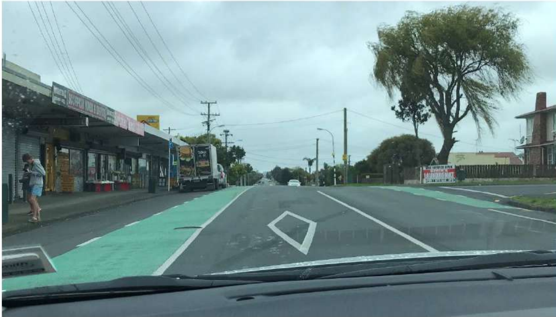
Figure 6: Inadequate sight distance to zebra crossing
